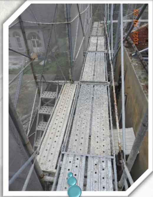
室外施工鷹架水平走道與上下樓梯錯開，增加行走搬運順暢及安全
