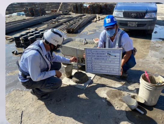
混凝土坍度試驗
