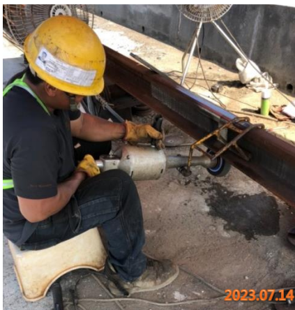
鋼軌底部研磨
